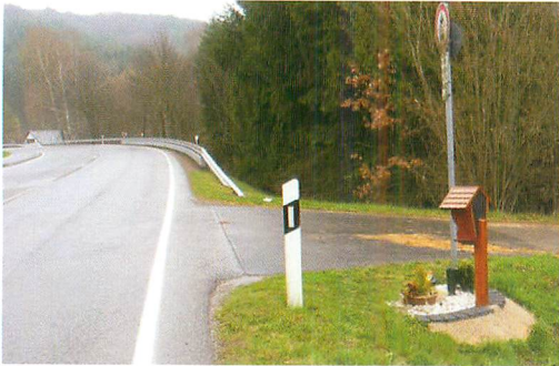
➤ Before: Critical junction in a bend.
