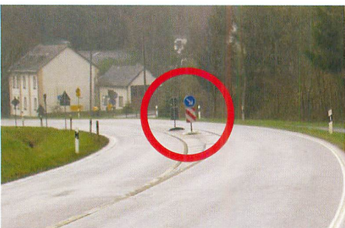
➤ Before: Median split with signs on steel poles.
