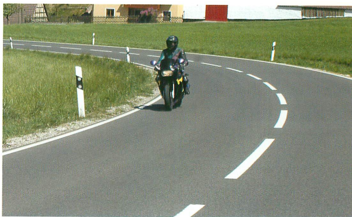
➤ Contiguous upgrading and rehabilitation of pavements to ensure even road tops.
