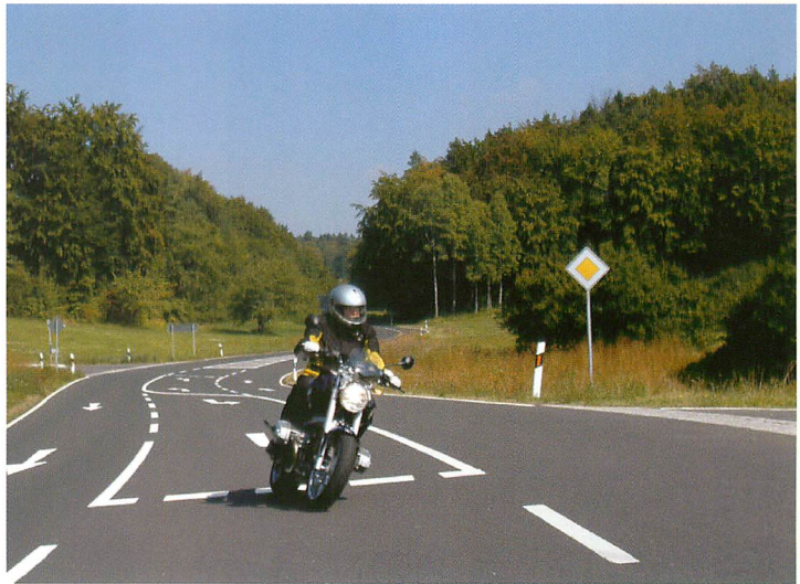
➤ Dedicated left-turn lanes create more safety.
