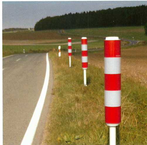
➤ The inexpensive flexible bollards have passed the real-life test.
