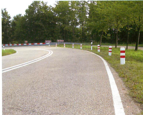
➤ “Balisette” test section on the “Schwarzwald-Hochstraße” (B462) in the Black Forest.
