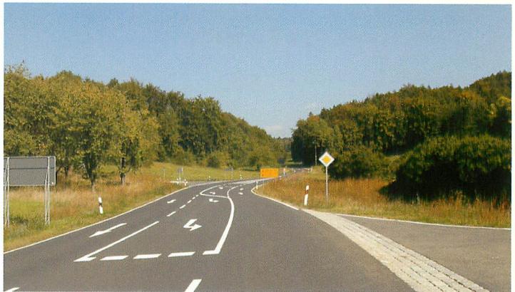
➤ Exemplary left-turn lane at a critical junction.
