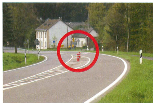
➤ After: Traffic signs were replaced with reflective flexible, red-and-white bollards.
