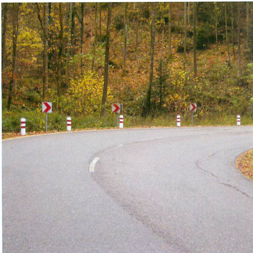
➤ Poor implementation of a good idea: red-and-white curve guidance signs are no longer necessary here.
