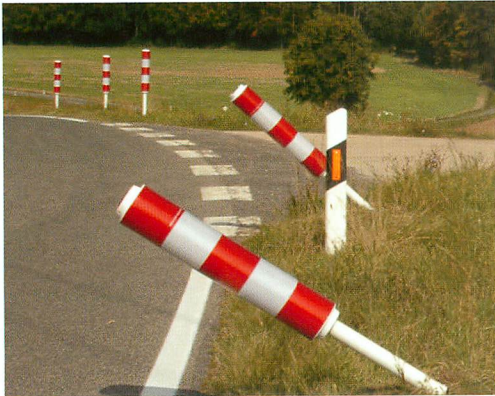
➤ Flexible bollards such as these are almost risk-free.
