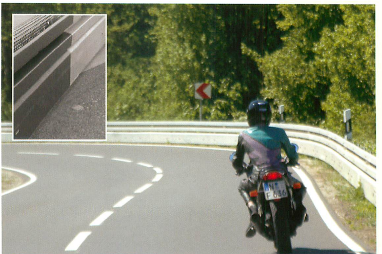
➤ The roadside on this curving road section has been secured by equipping guardrails with underrun protection (“Euskirchen Plus” system).
