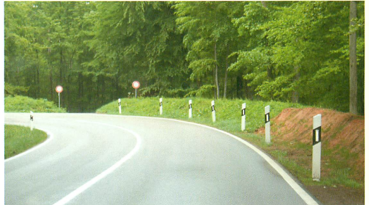
➤ Making the outside bend more forgiving in critical sections by installing earth berms.
