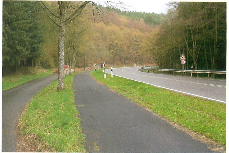
➤ Before: Long tree-lined bend with rigid steel sign-posts (obstacles on roadsides).
