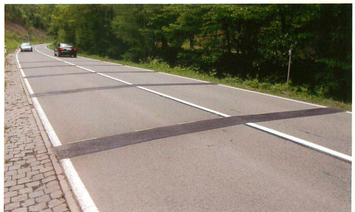
➤ Rumble strips (asphalt, raised approx. 1.5cm; 50cm wide) are an effective way to make motorists slow down.
