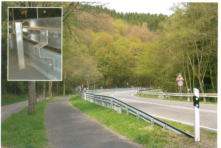
➤ After: New crash barrier equipped with underrun protection to prevent collisions with obstacles, cyclists and pedestrians.
