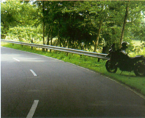
➤ Curvy road without underrun protection.
