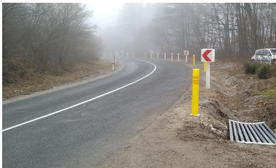
Figure 33: Example of best practice with appropriate indication of curve and junction with other safety elements for motorcyclists (source: R. Strah).
