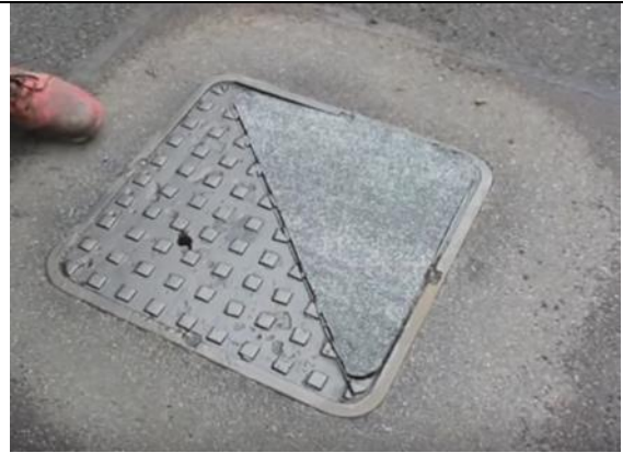
Installing special anti-skid drain covers (Source: Geveko Markings)
