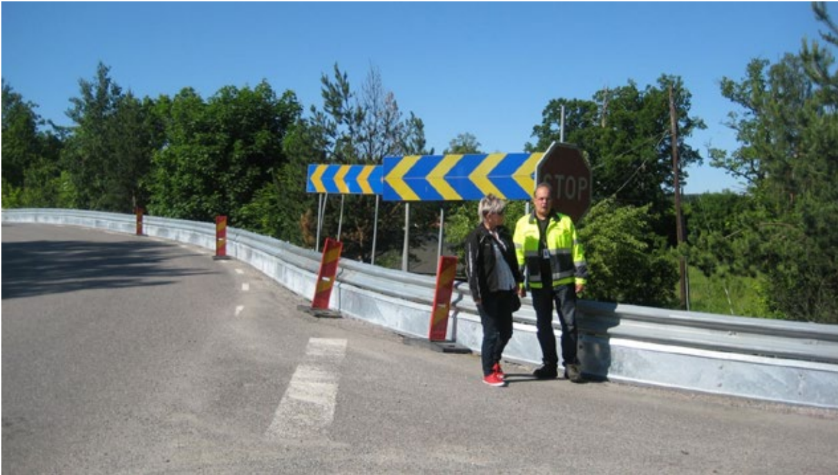
Picture 4. The first barrier with MPS was installed on a road outside Åkersberga May 2012.
