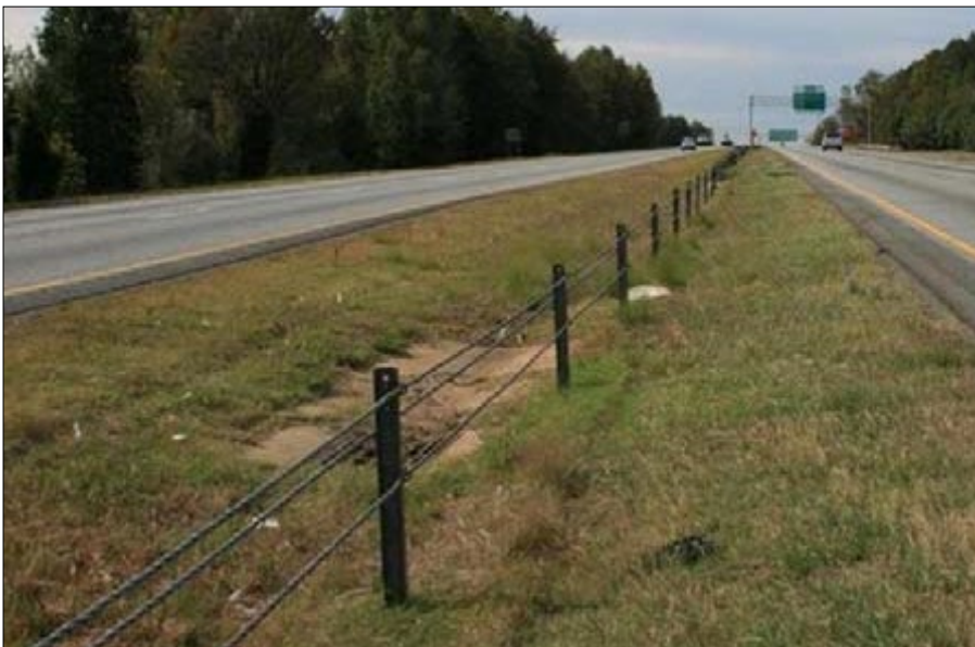
Picture 1. Median cable barrier installation in USA
