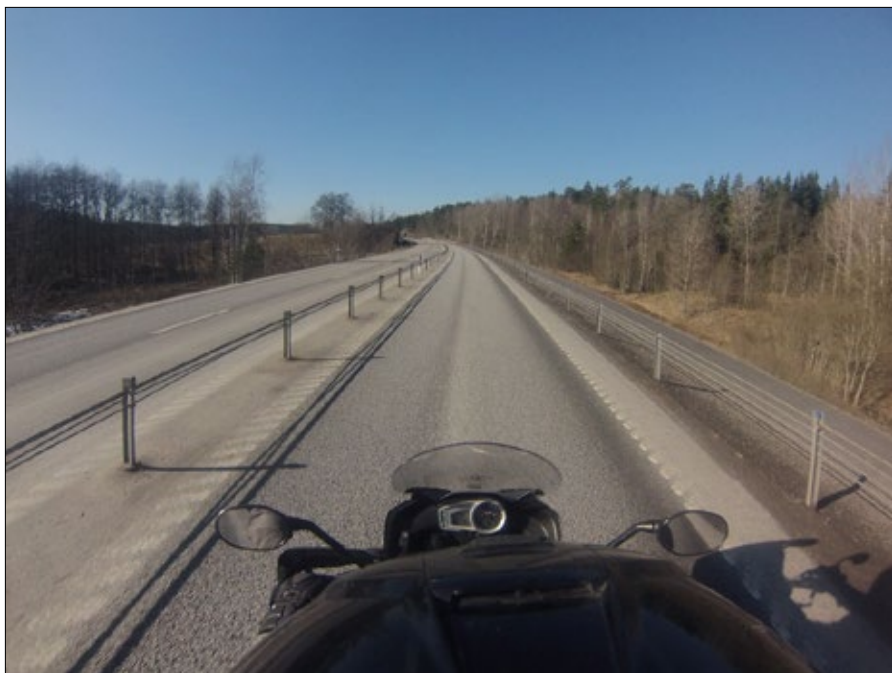
Picture 2. Cable barrier installation 2+1 in Sweden (Finspång-Norrköping).
