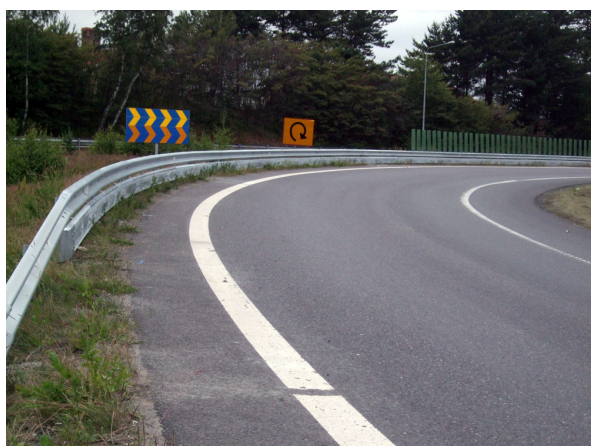
The same exit with new guard rail and motorcycle protection system installed
