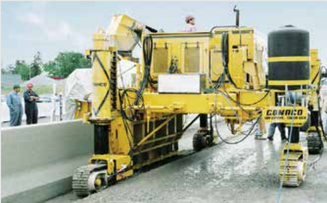
Picture 5 - slip formed concrete barrier
