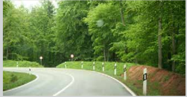
Picture 18 - Earth walls replacing guardrails
