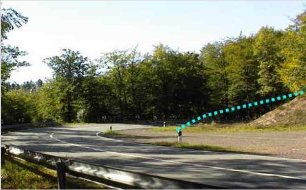
Picture 19 - Obstructing view cleared, reducing the risk of run-off and/or frontal collision
