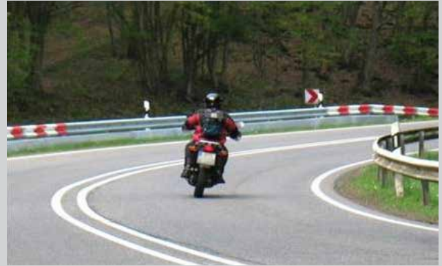
Picture 20 - Double continuous line to reduce the risk of run-off in curves
