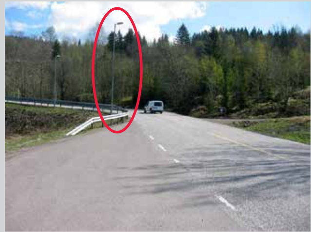
Solution : clear trees, move light post to the inside of the curve
