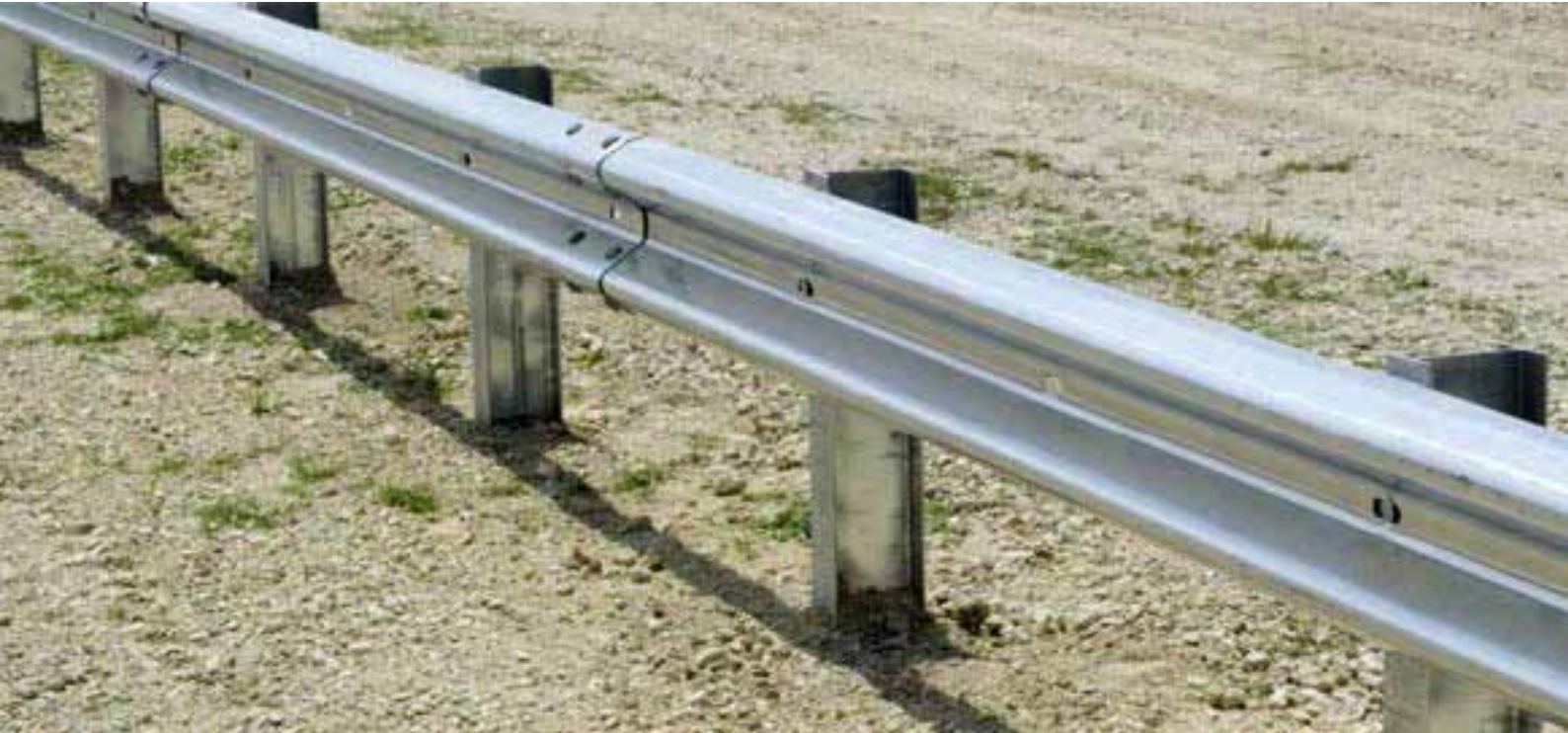
Picture 3 - normal steel guardrail
