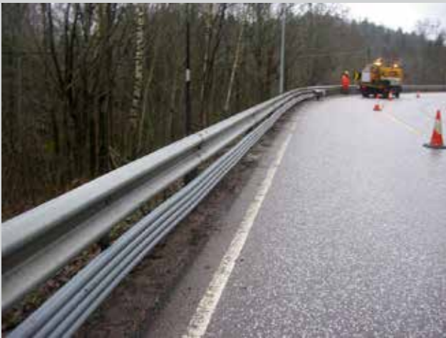
Picture 22 - Polyethylene subrails have been added to guardrails in outer curves.
