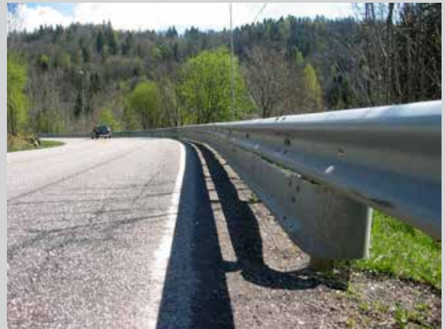
Picture 23 : Motorcyclist-friendly steel subrails have also been added.
